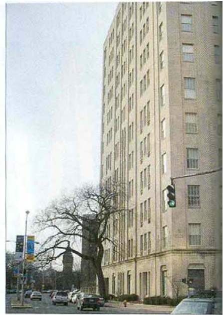
With spectacular views of Bushnell Park and Downtown Hartford, the former SNET building on Trumbull Street has been transformed into 132 upscale apartments.
